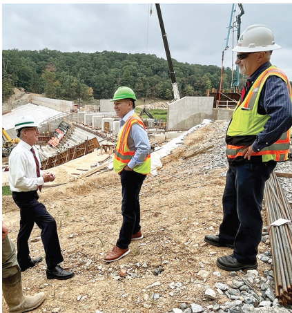
Congressman Lloyd Smucker tours Lake Williams Dam, the largest infrastructure project in York County.
